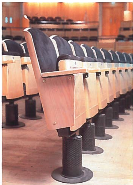
Stall seating, with pedestal air supply!
