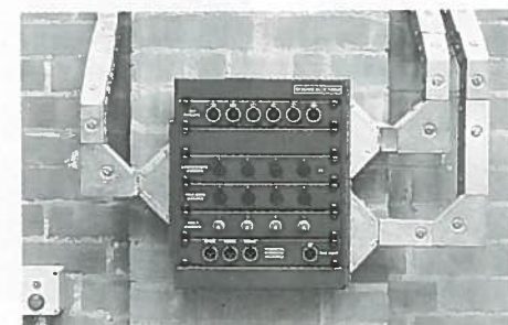
The side stage sound outlet box.
