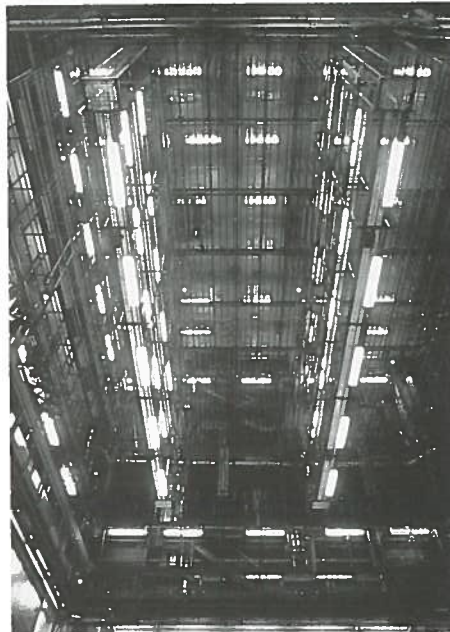
Looking from the stage to the grid, showing two of the three lighting bridges and back lighting gantry.
