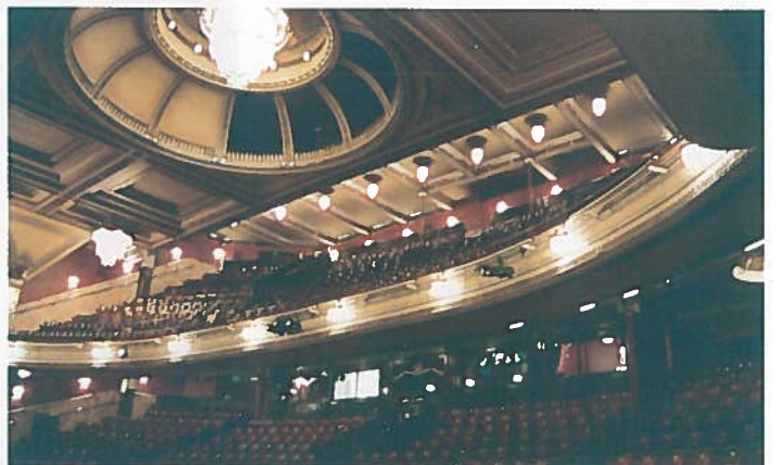
New lighting positions have been created through installing catwalks above the dome. Eight motorised ceiling panels allow the voids to be closed when the house lights are on.
