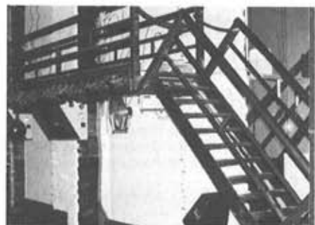
The hinged stairs allow access from the side walkways from the balcony directly on to the stage area when no performance is taking place.
