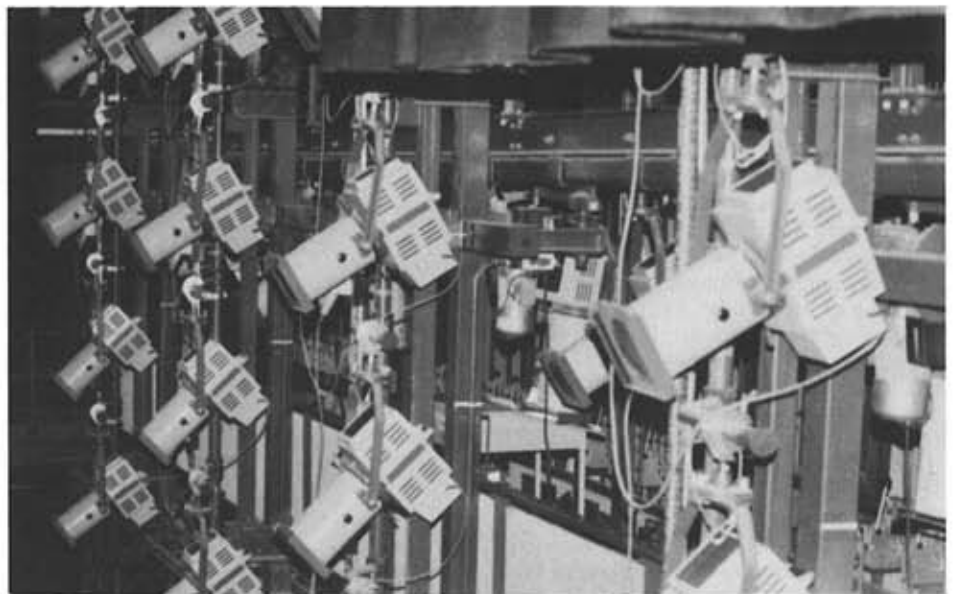
Spotlights on the side bridges are on motorised drives, shown in detail below.
