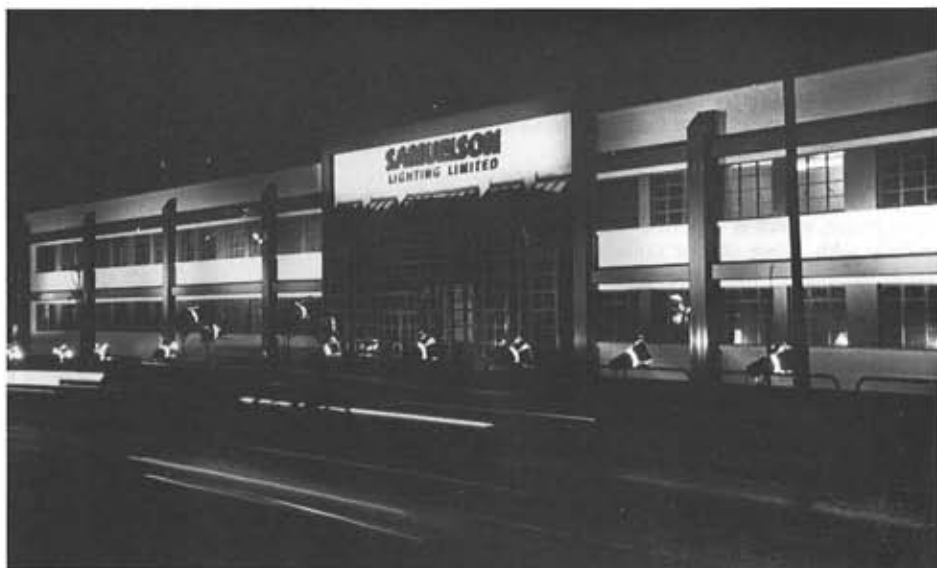
The newly renovated facade at Samuelson Lighting's North West London headquarters, Samcine West.
