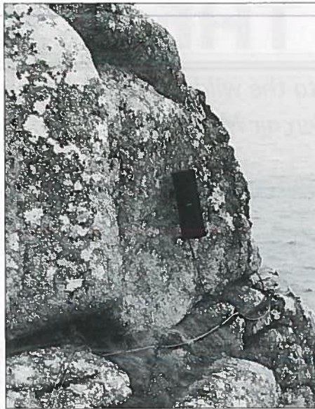
One of the Bose speakers rigged for action. All the speaker and lighting cable runs are armoured and all equipment is RCD'd.
