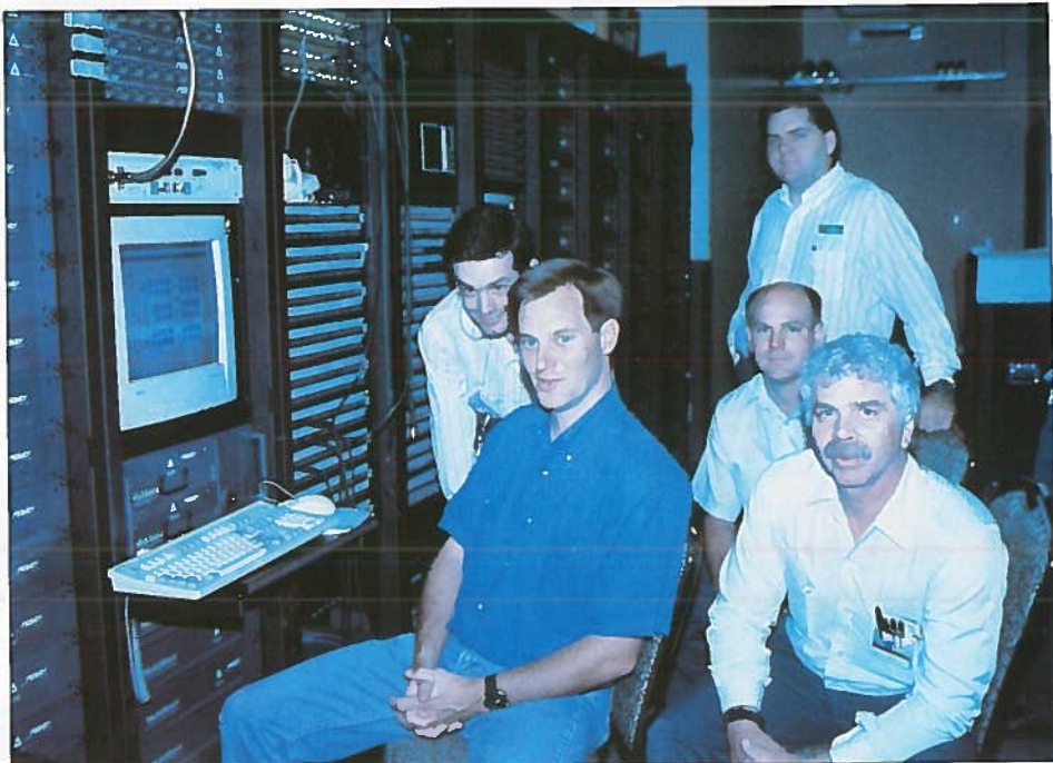
System designer Vance Breashears of Sound Technology Consultants (in blue shirt, second left) at the NexSys workstation in the Main Control Room, with members of the team from the Opryland audio video crew.
