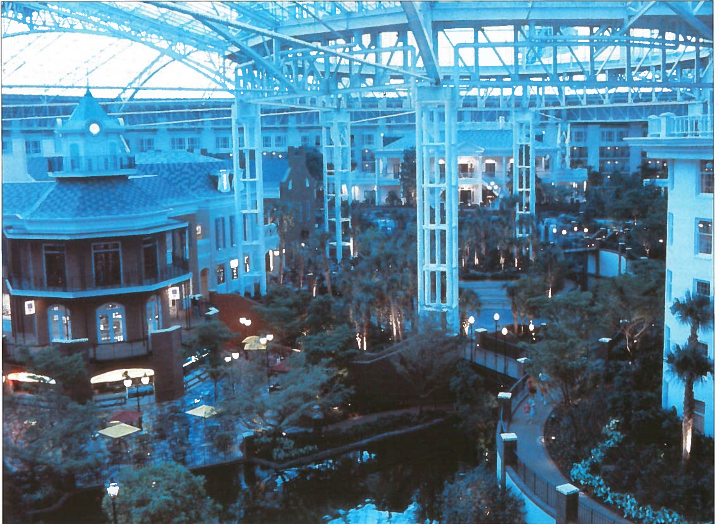
The vast Delta, a 4.5 acre development fully landscaped housed beneath a soaring 15-storey high glass dome weighing 650 tons. A river, waterfall, eight retail shops, six restaurants and ante-bellum mansion make this themed space a 'destination' in itself.
