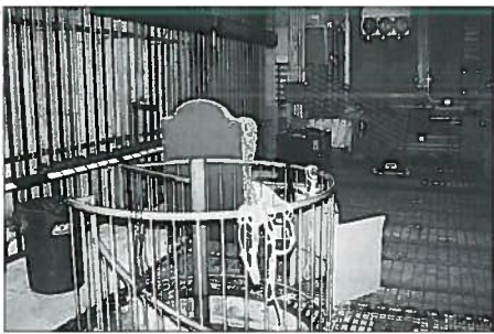
The Geary's fly floor, showing the mesh floor and spiral staircase.
