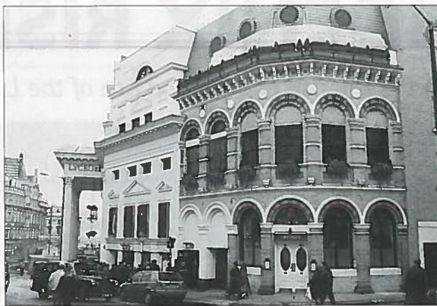
The new wing to hold dressing rooms as well as bars, hospitality suites and a restaurant, appropriately named Irving's.
