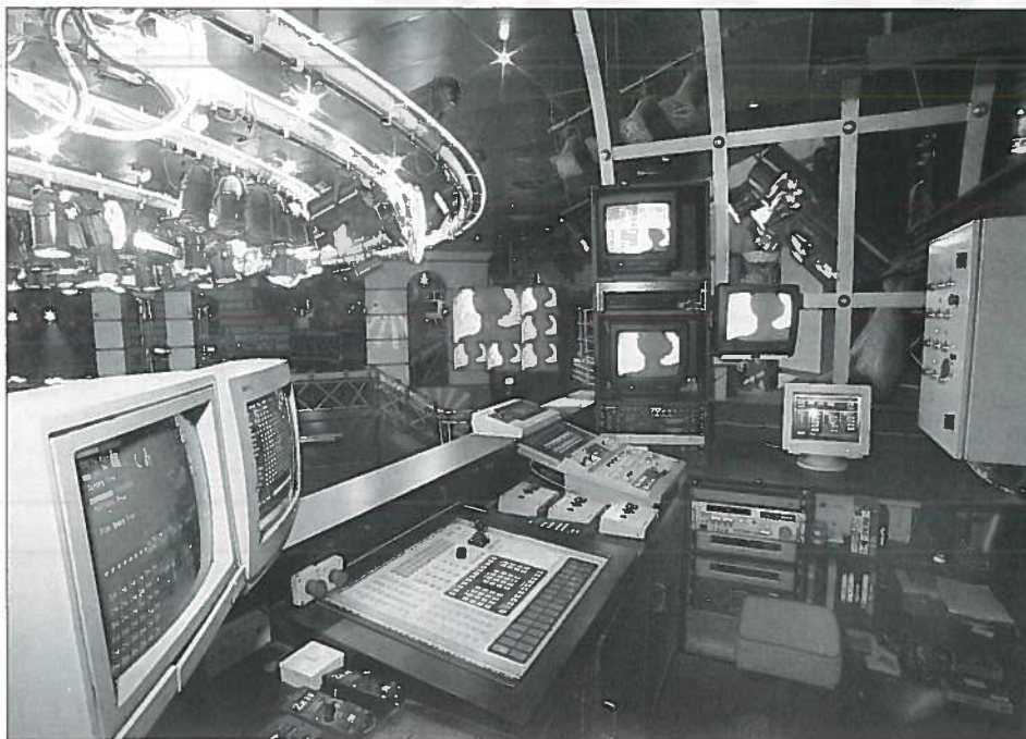
The main control area awash with technology.
