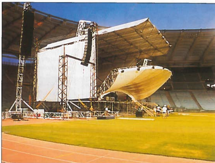
The Total Fabrication PA towers for the V-Dosc system.
