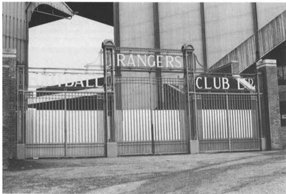
Main Stand/Govan Stand entrance at Ibrox Park.
