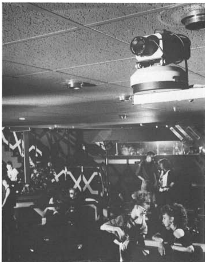
One of Toa's CCTV cameras installed adjacent to the dance floor at The Palace, Blackpool. The camera contains an auto-iris and is mounted on an autopan base.
