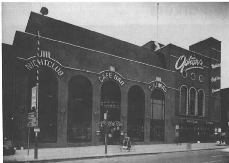
The completed Granada 'Options' complex at Kingston Upon Thames. Similar Granada mixed media venues are expected to follow.
