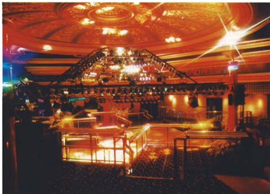
The lighting rig at Options, Kingston is supported by three pillars, leaving the splendid ceiling untouched.
