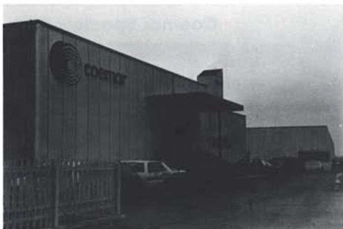
Coemar at Castel Goffredo. The new building can be seen in the background.
