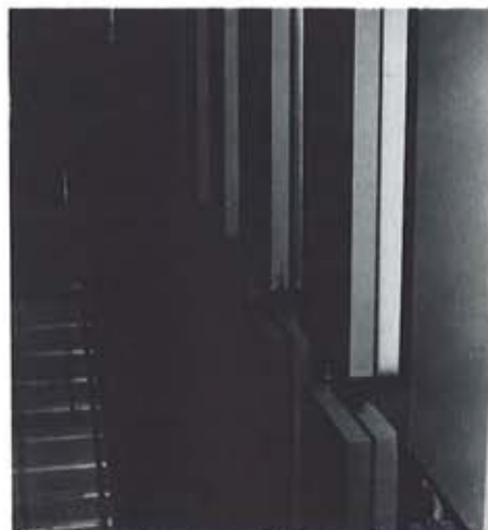
Hinged panels on the auditorium walls can swing round and open like a book to alter the acoustic.
