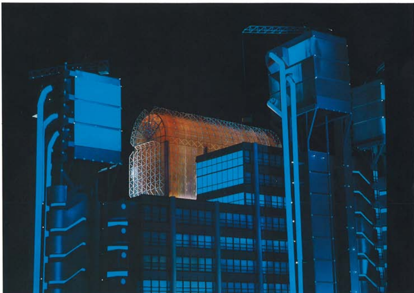
The main body of the Lloyd's building has been washed in blue light with white beams for lift shafts. The 200ft central glass atrium was separately treated, lit from both inside and out in a golden rosy amber and pink.
