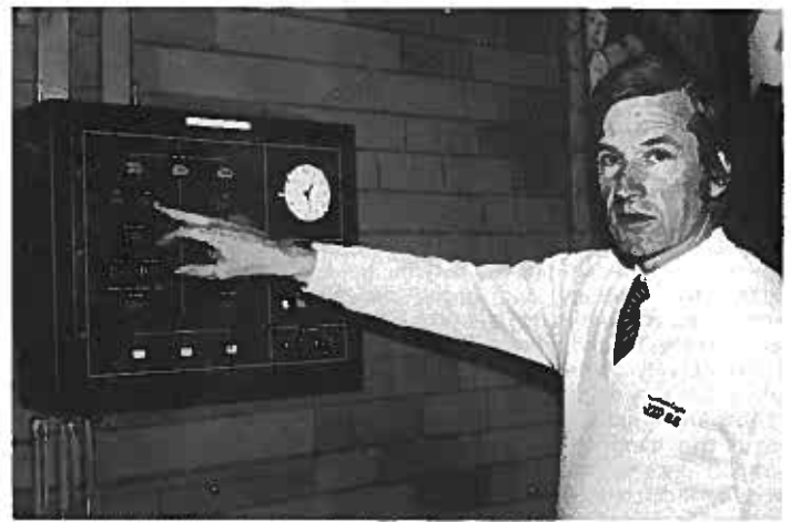
Northern Light's Mike Smyth with the System 2000 working light control.
