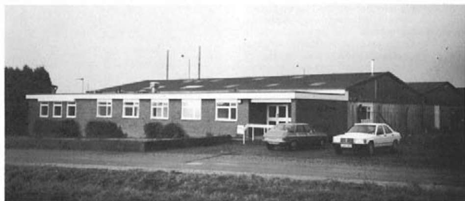
H.H. Electronics' new Huntingdon factory.
