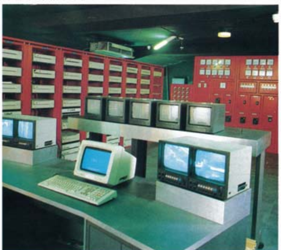
The control room: around the desk are video monitors which look at pictures from 27 cameras placed through the museum. The technician even has a video display giving information on the state of the air conditioning within MOMI.
