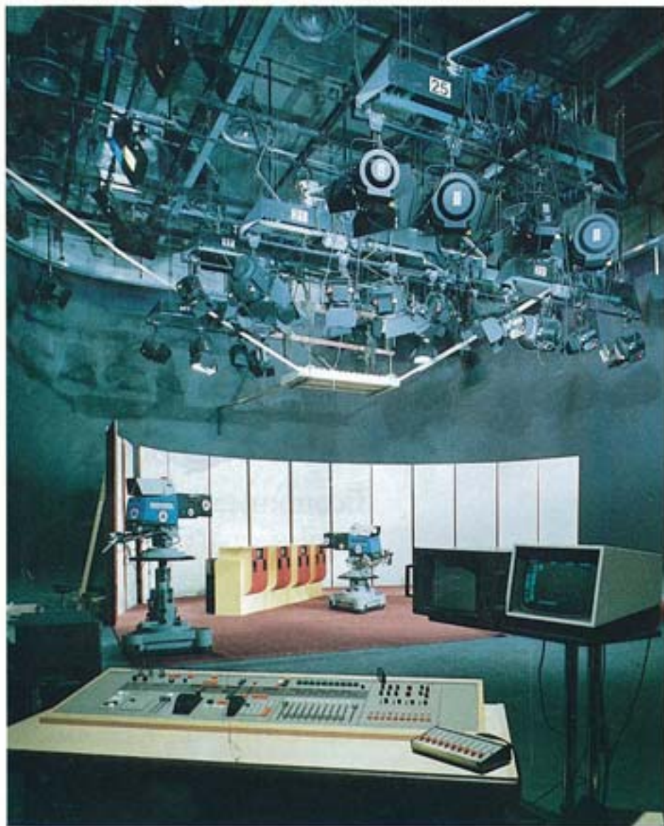
Studio 'La 5' - a private TV studio in Paris. Luminaires are Quartzcolor and control is by a Strand 96 channel Gemini.
