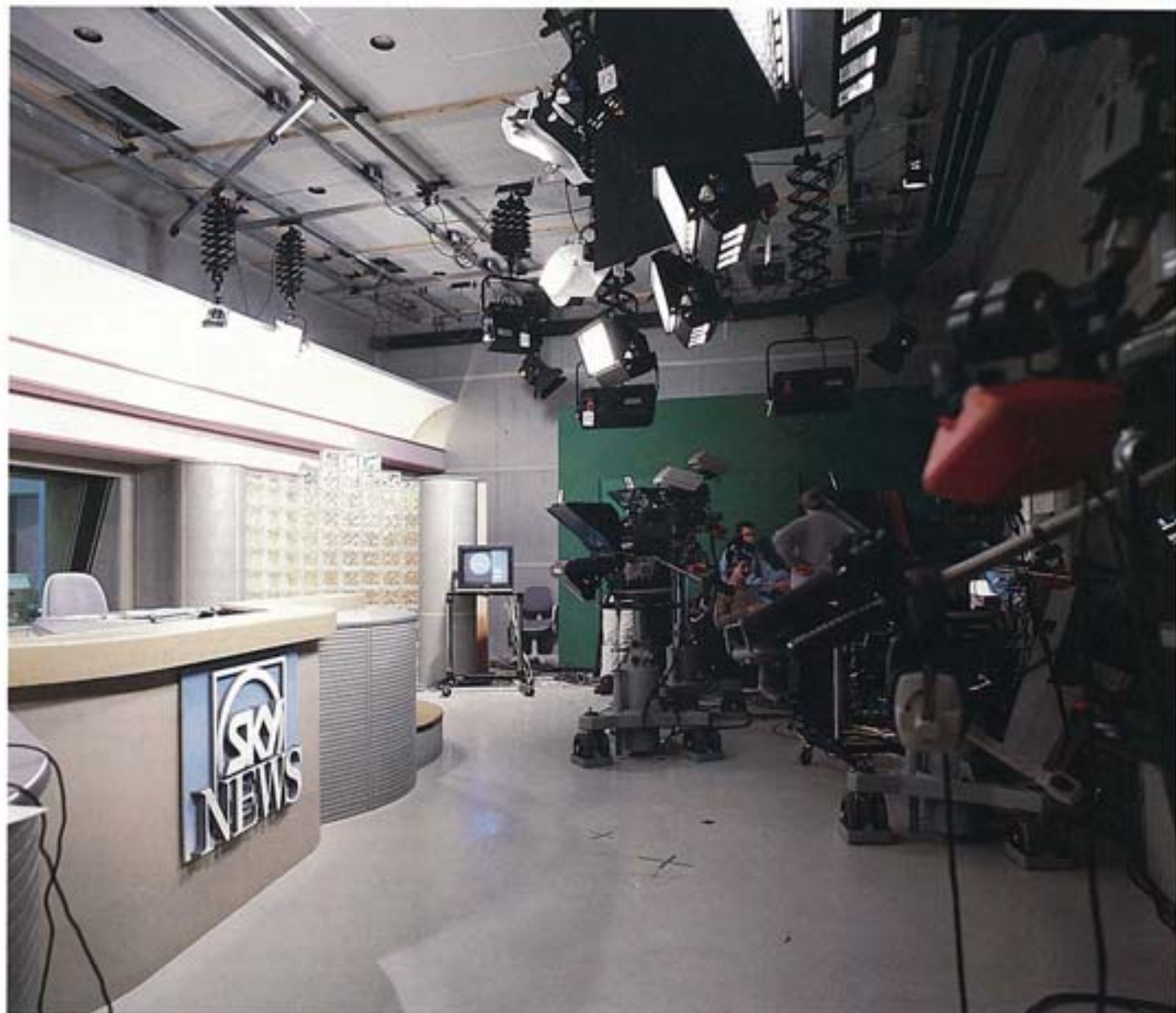
The news studio at Sky Television with everything in place bar the readers. The lighting rig gives complete flexibility of position and height for each lantern. Equipment supplied by Strand Lighting to Sky includes Mizaris, Polaris, Castors, Artusos, Softlights, Iris 2's and Mini Irises. Strand also supplied 14 ENG kits with Redheads and Blondes and battery kits.
