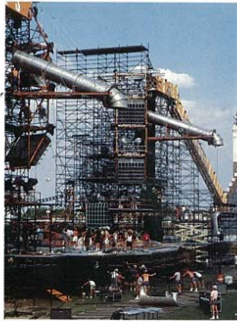
The lighting rig features the largest colour changers in the world, measuring 8ft x 4ft. Forty are in use on the tour and they were custom-built by Light & Sound Design of Birmingham and supplied by Presentation Consultants Ltd. In addition, 88 MoleMags and 100 ColourMags were used.
