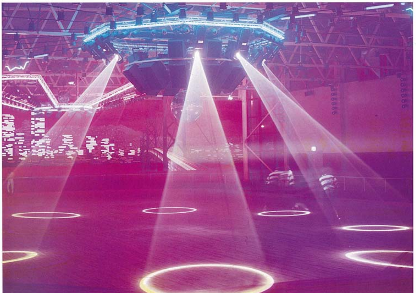
The central loudspeaker cluster consists of 12 Turbosound TMS-5 loudspeakers in a single ring augmented by six TSE-11 mid-high packs.
