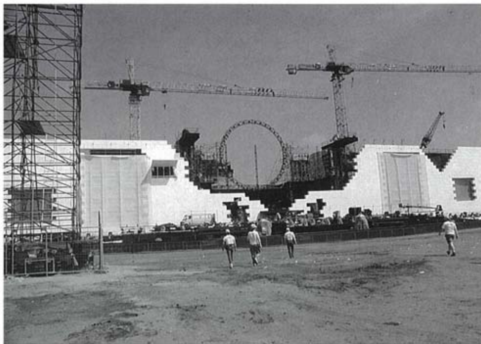
The Wall goes up.
