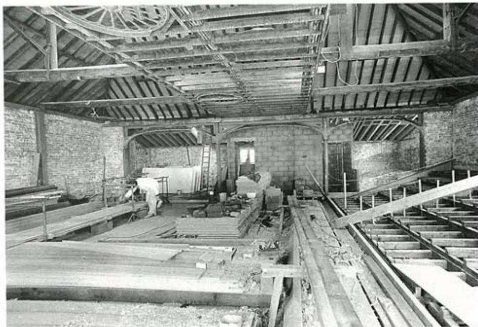
Mid-term construction underway.
