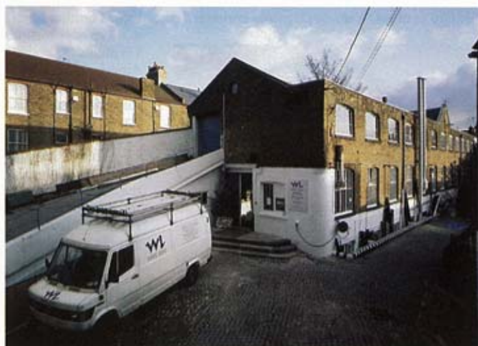
Part of White Light's Fulham base. Ever more activity is being shoe-horned into the site.
