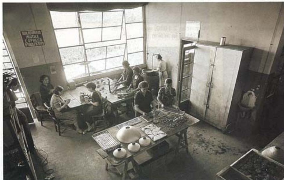
Part of Coemar's original factory in Milan - note the spun reflectors.
